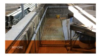
Access to the air cooling towers has no designated walkway and there are trip and electrical cable hazards. There is also no clear delineation between the walkway and the "no step" areas on the cooling towers.
