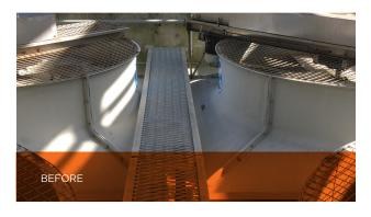
Existing walkway is too narrow to be safetycompliant and provides inadequate protection from the risk of falling onto the cooling towers "no step" area. Access to service areas is difficult.
