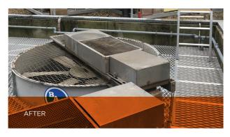
The new raised work platform eliminates trip and electrical hazards. There is safe way to access motors and other maintenance areas across "no step" areas. The walkway has non-slip texturing.
