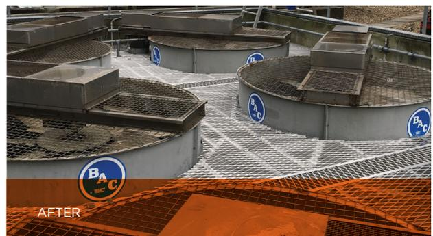
New, raised walkway provides a safe and even platform for accessing the cooling tower area.
