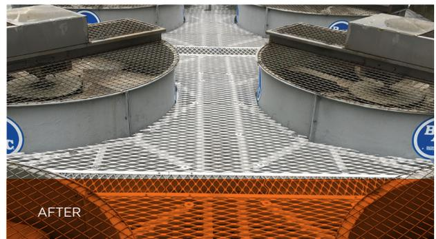
Raised platform eliminates the fall risks and provides a safe and even surface for working on the cooling towers.
