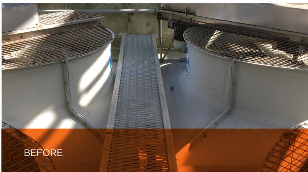
Existing walkway is too narrow to be safety-compliant and provides inadequate protection from the risk of falling onto the cooling towers “no step” area. Access to service areas is difficult.
