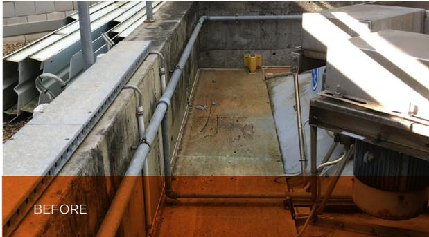
Access to the air cooling towers has no designated walkway and there are trip and electrical cable hazards. There is also no clear delineation between the walkway and the “no step” areas on the cooling towers.
