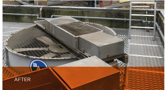
The new raised work platform eliminates trip and electrical hazards. There is safe way to access motors and other maintenance areas across “no step” areas. The walkway has non-slip texturing.
