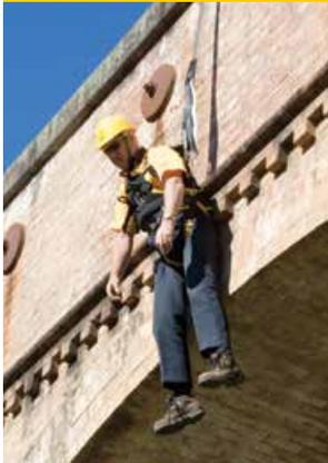
**5** Fallen worker with Shock Absorbing Lanyard removed
