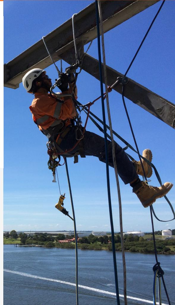
**The Tower Workers harness** comes equipped with forward rings and a drop seat or buttock pad. This is designed to hold the user in position to allow hands free work for extended periods of time. It is ideal for all tower or pole work.
