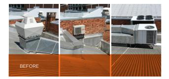
Roof access to the air conditioning units. Anyone accessing these units would have difficulty moving about due to the roof slope and could slip, damaging the roof, or injuring themselves.
