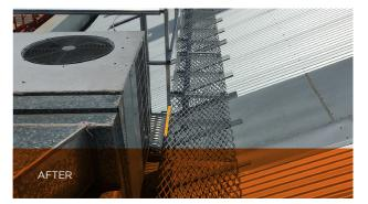
Raised walkway provides safe maintenance access and an even working platform across the entire cooling tower area.
