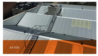
A walkway and raised platform eliminates the fall risks and provides safe access to the aircon unit.
