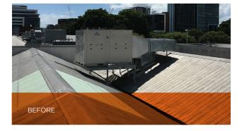
Aircon unit lacks any platforms and roof access goes past skylights that are considered a fragile surface and which pose a fall risk. It is likely that repeated maintenance trips will result in roof damage.
