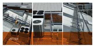
Raised work platform eliminates all hazards. There is now safe access to the motors and other areas that require regular maintenance. The walkway non-slip.
