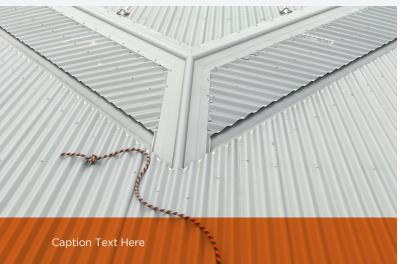
We relocated these anchor points to a position that would guarantee proper performance and structure integrity while still allowing safe, roped access to the entire roof area.
